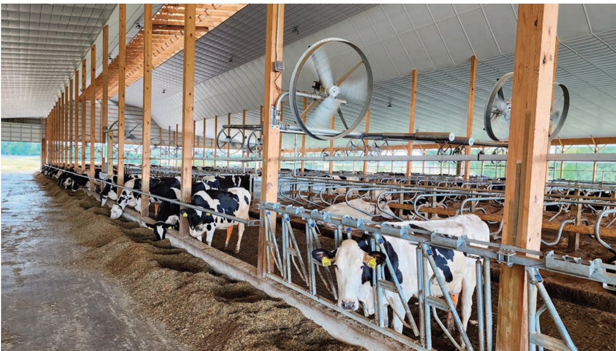
Unlike many free-stall barns, the new main barn at Walton Farms features nine rows. Despite its immense size, the 36.5-foot high peak of the paneled ceiling creates a natural draft while fans also help to exhaust stale air. Note the slope of the
