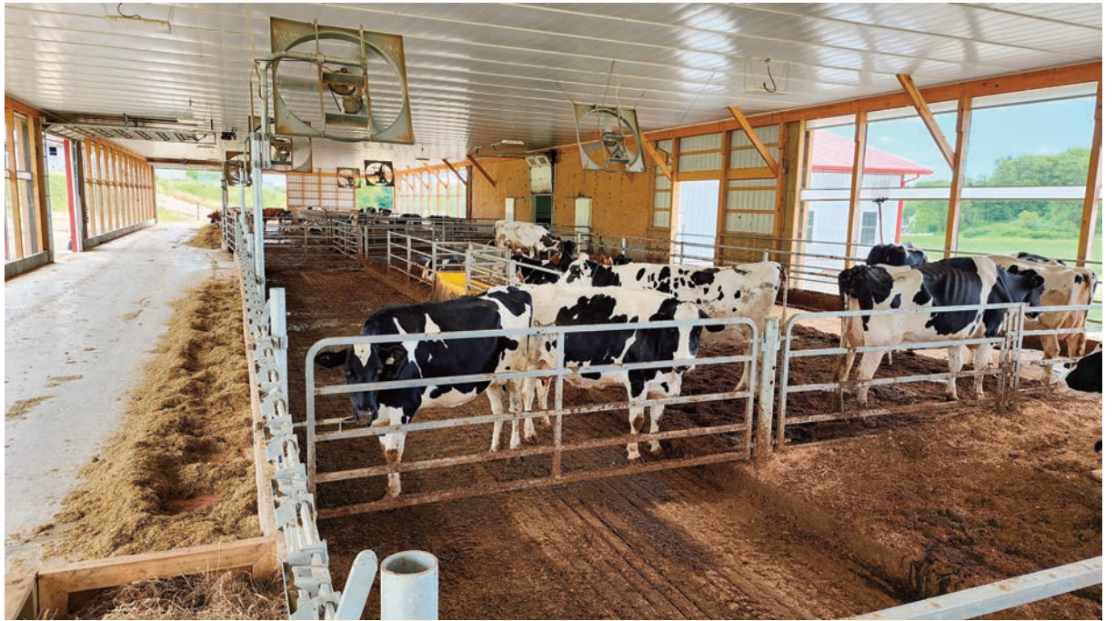
Most noteworthy about this picture is that there are two manure alleys ... one where the cows are standing and the other on the far side. In between those two lanes are the box stalls (near) with freestalls in the distance. The wide feed alley makes for easy and efficient delivery of rations. Nothing in the barn is automated.
