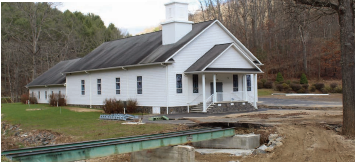
A church in Lansing, N.C. stands amidst clean-up efforts following Hurricane Helene.
